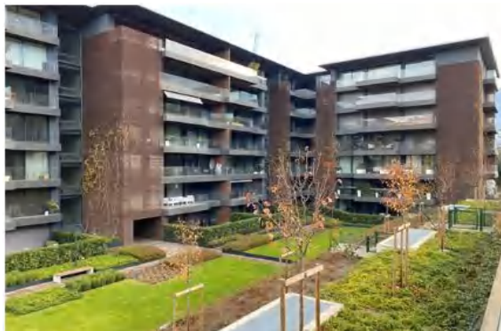
Parcolago apartment in Switzerland
